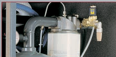
EXTERNAL SPIN-ON AIR/OIL FILTER SEPARATOR Quick to replace.
